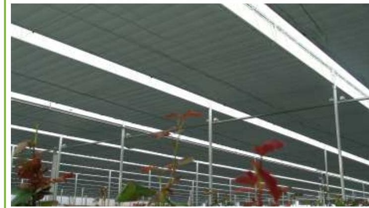
Thanks to this system, it is possible to control the climate and energy consumption inside the greenhouse. In the built-in PUSH PULL curtain, special aluminum tapes are used to prevent harmful sunlight from entering the greenhouse and to maintain warm air in cold weather.
